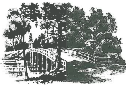
OLD NORTH BRIDGE
